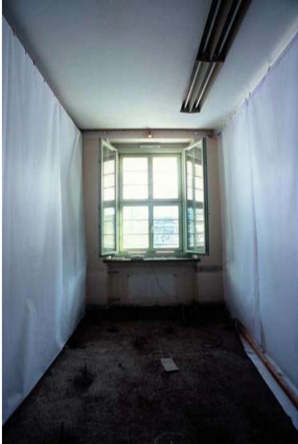
exterior upper window: daylight redirecting glass “Okasolar W”; exterior lower window: electrochromic glazing; interior window: double low-E
